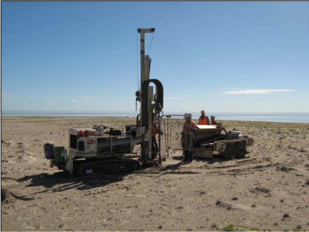
Figure 23. Point Sturt site during piezometer installation showing absence of cracking (from Earth Systems 2008).
