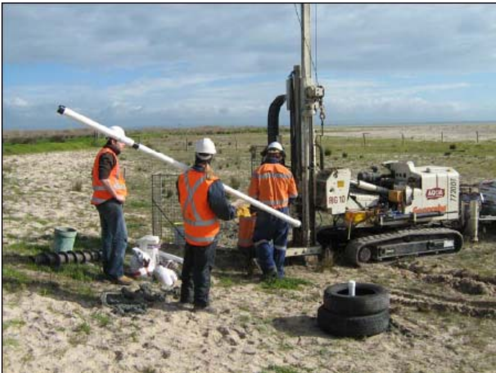
Figure 22. Campbell Park site during piezometer installation showing absence of cracking (from Earth Systems 2008).
